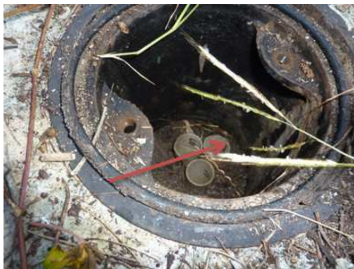
Figure 7 For monitoring wells it was always measured the position of the top of PVC pipe 1
